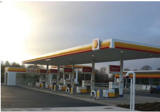
The Global-MSI canopies, sales building and car wash building, Livingston, built for Shell in 2011
