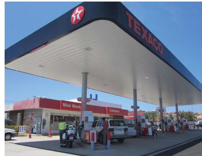
The Global-MSI canopy built for Chevron Espana San Bartolomé de Tirajana, Gran Canaria in 2011
