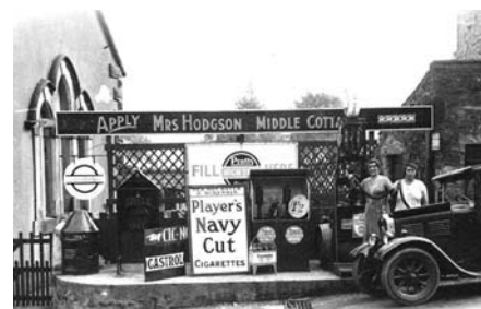
Kerbside petrol from 1930's
